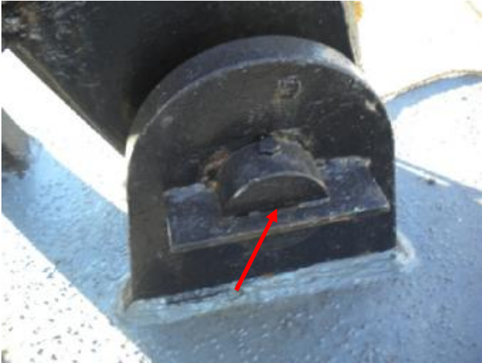
Fig. 6 – Transom Reference Point Stbd Side
